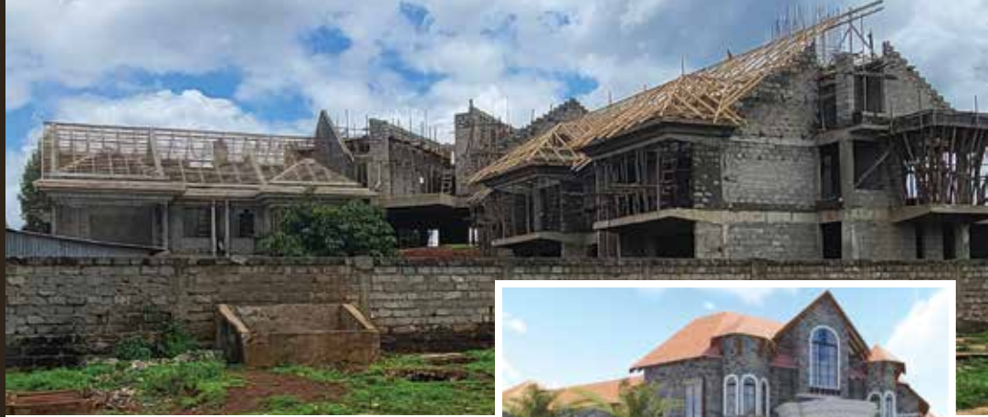
(above) Construction progress on Ambatana Manor as of May 2023
